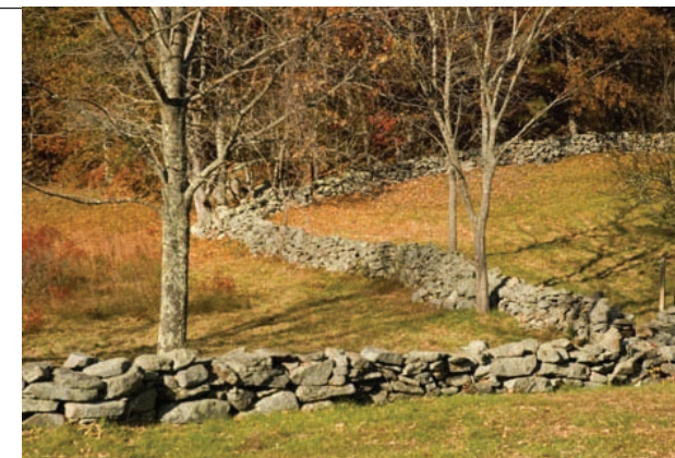
Carefully laid stone walls have survived hundreds of New England and New York winters, even as cement walls crumbled and disappeared.
